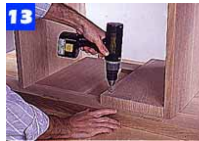
The drawer blocking is made from two pieces of plywood with solid oak facing. Screw the blocking to the case side.
