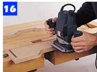
Cut out the profile on the top edge of each drawer front. Next, use the router to cut the cove along the edge.
